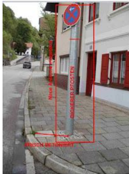
Figure 3: Example of 5G pole in Germany (source: a friend in Germany).
