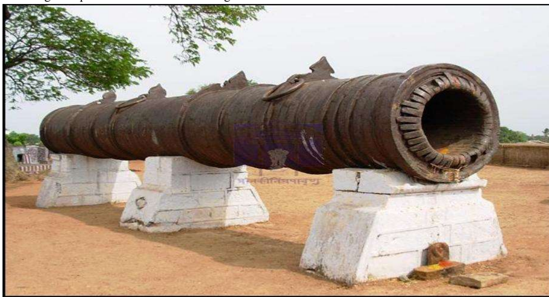
17 th Century forge-welded iron cannon in Thanjavur, Tamil Nadu (source: CAG report 2013)
