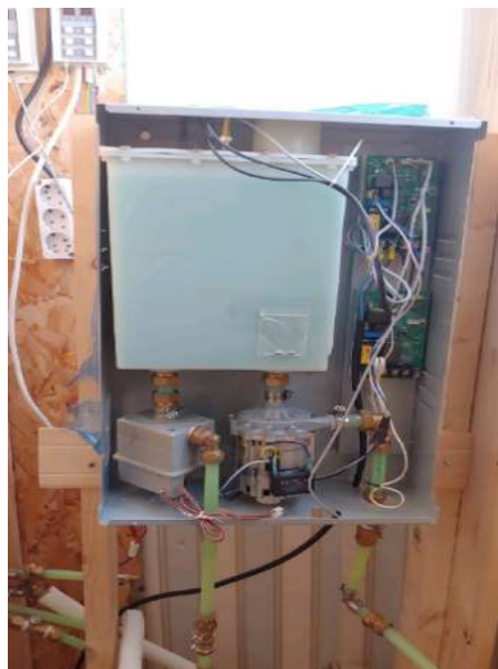
[Fig. 3] Integrated water bath boiler for supplying hot water heat to mobile home
