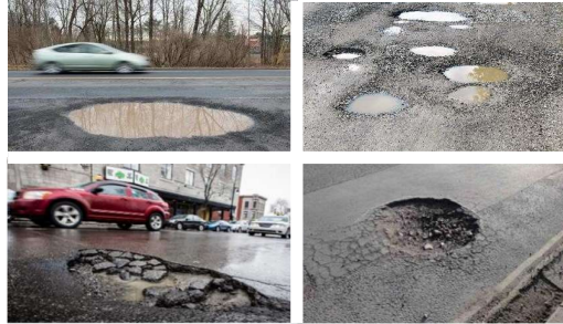
Fig.1 Sample potholes from the dataset
